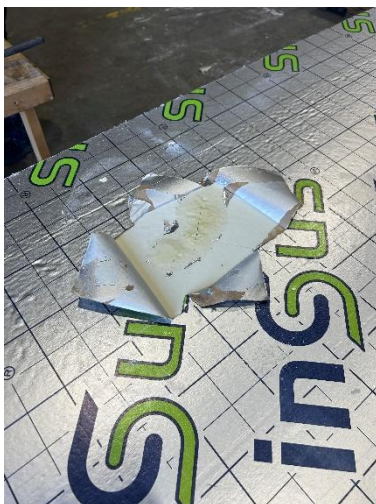
Picture 39 insulation after testing
