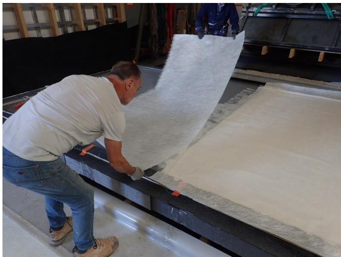
Photo 9 The reinforcement is applied.
