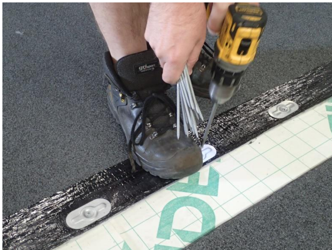
Photo 4 The roof waterproofing sheet is fastened.
