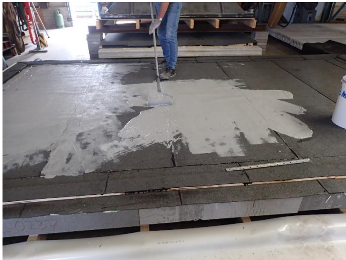
Photo 8 The primer is applied.
