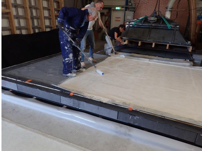
Photo 10 The coating is applied.
