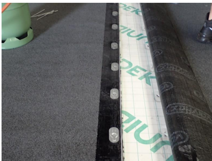
Photo 5 The fastening system has been placed.
